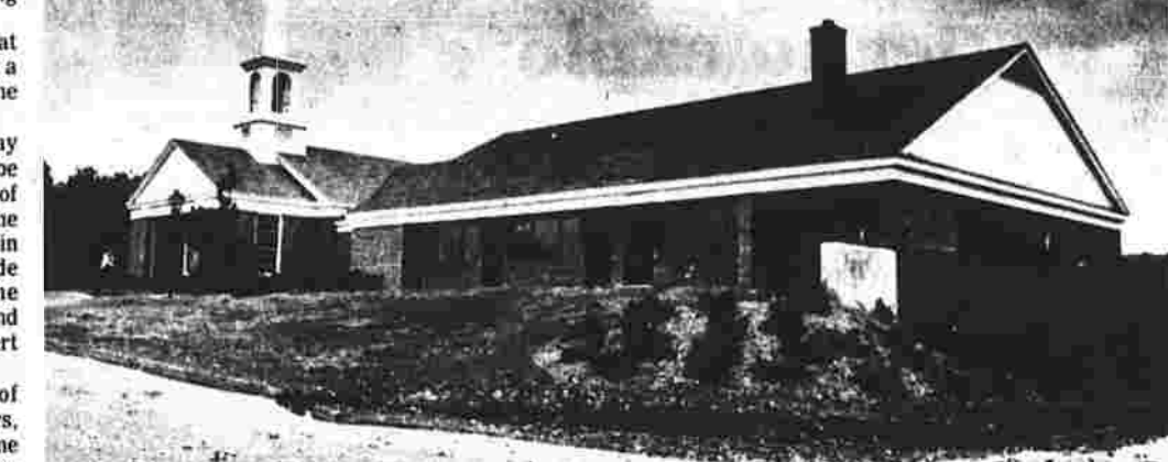
This is the Trinity Congregational Church on Hackmatack Street as it looks with its newly completed educational wing. (Herald photo by Pinto)
